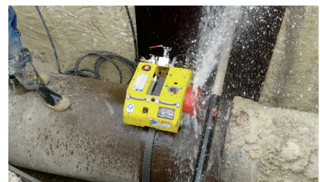
Severing a water pipe under pressure, the Trav-L-Cutter stays on track
