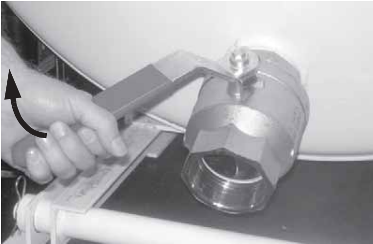
Figure 3-20. Close the tank drain valve when the liquid has finished draining.
