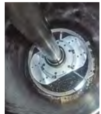
Internal cutting module lowered to cutting depth
