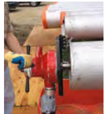
SDB pipe end preparation
