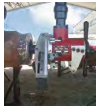
SDB end prepping pressure vessel
