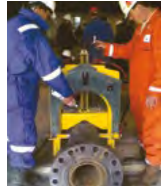
Guillotine cutting pipe
