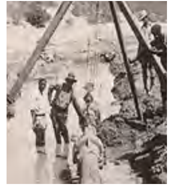
Early pipe fitting
